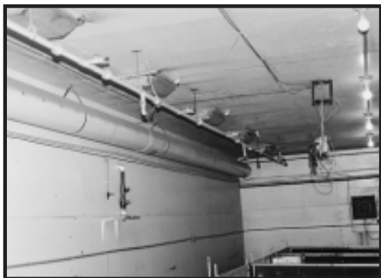
Oil sprinkling system installed in a commercial room at PSCI.
