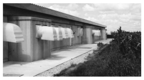
*Figure 1:* Fan arrangement and manure pit design along the sidewall of the concrete barn built by *FRED GROENESTEGE CONSTRUCTION LIMITED (Sebringville, ON).*
