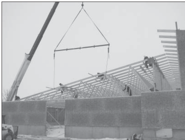
Construction of the new facilities at Prairie Swine Centre (Floral) will provide an opportunity to update aging facilities
