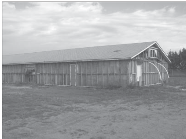
Barn 7 in early demolition, previously used for gilt development
