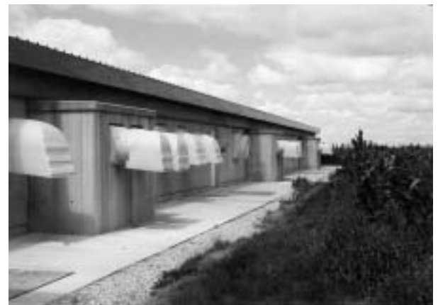
Figure 1 Fan arrangement and manure pit design along the sidewall of the concrete barn built by FRED GROENESTEGE CONSTRUCTION LIMITED (Sebringville, ON).
