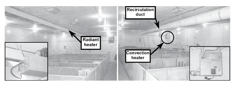
Figure 1. Photo of the experimental rooms. A: Treatment room with a 50-ft long infrared radiant heater (inset- heater part); B: Conventional production room with a forced-air convection heater (inset).
