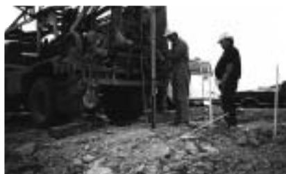
PFRA installing piezometers.
