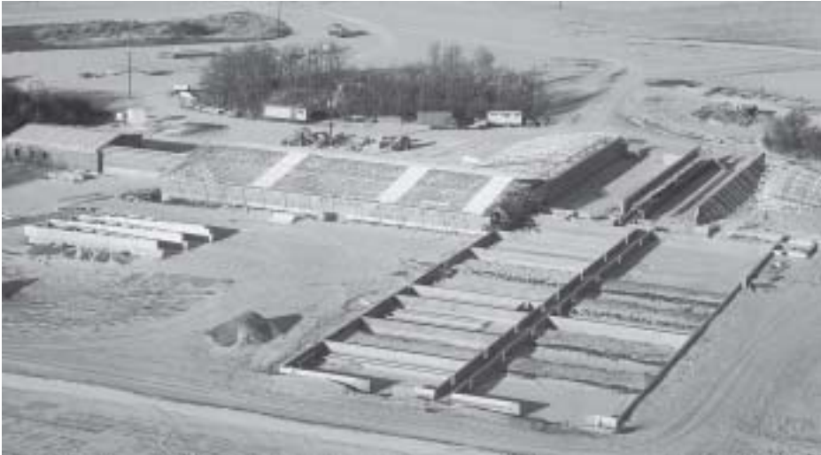
Aerial photo of 600 sow facility under construction Above photo taken December 21, 1999
