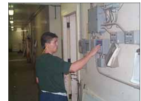
Reducing temperature set-point can increase growth rate 2-5% during summer months
