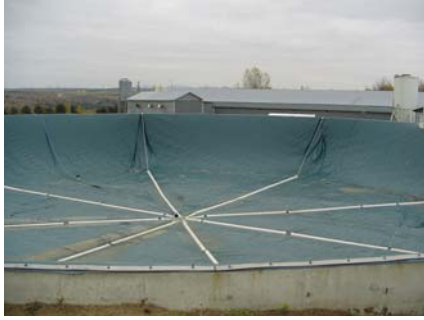
A manure storage cover near Sherbrooke, QC significantly reduces manure odour, rainwater dilution and conserves valuable crop nutrients
