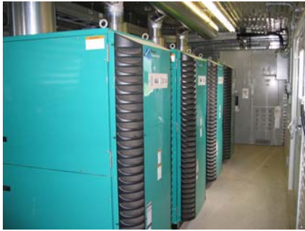
Four Capstone micro-turbine engines operating on methane produced from liquid hog manure in Saskatchewan. Turning methane into electrical energy will likely be a practice capable of netting carbon credits.
