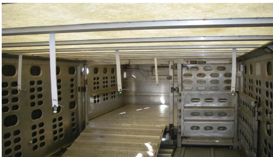
Figure 1. Placement of data loggers in the trailer (compartment 3).
