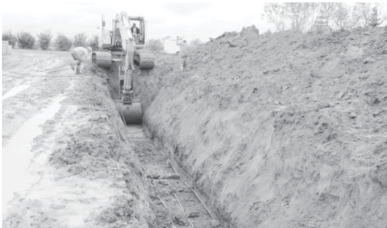
Figure 2. Installation of pipes for the ground source heating system installed in a grow-finish room.
