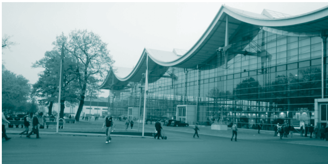
One of the 26 buildings housing displays at Eurotier 2014
