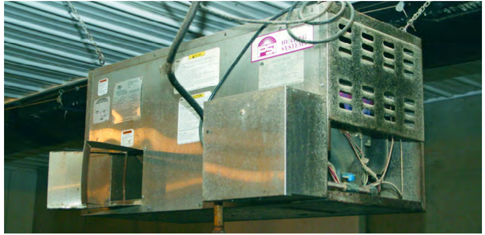
Having more furnace or heater capacity than required leads to more variable temperatures and higher energy bills
