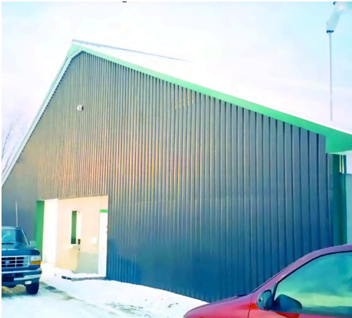
A Solag panel wall on a hog barn, which can increase incoming air temperature by 8-10°C
