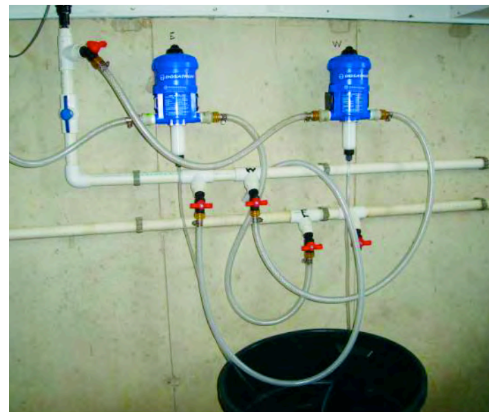
Two medicators for 2400 wean-finish pigs with 125 litre (33 gal) stock solution reservoir
