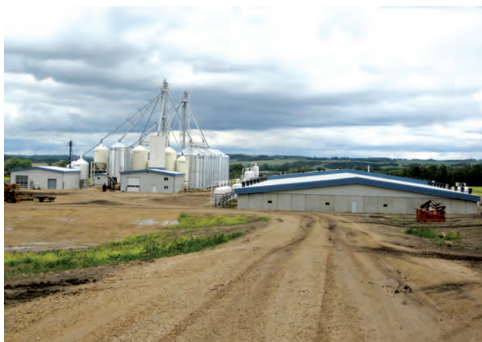
The new 800-sow hog barn and feed mill at Hartland Colony
