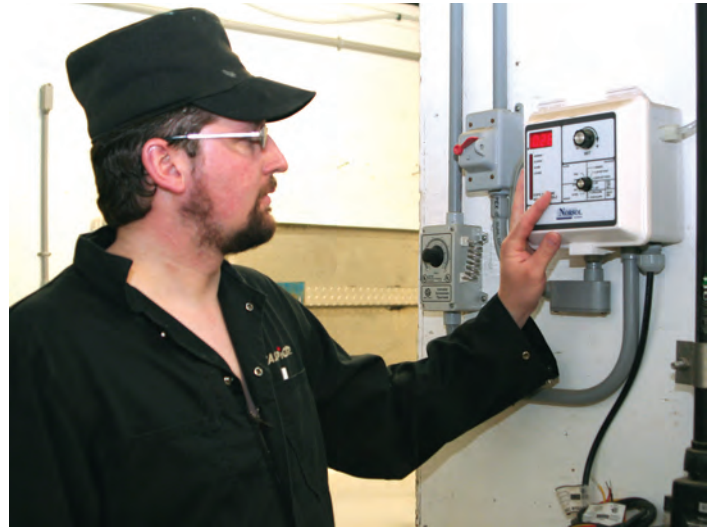
Martin Waldner, Hog Boss at Hartland Colony, adjusts the computerized environment controller for one of the nursery rooms continued on page 20
