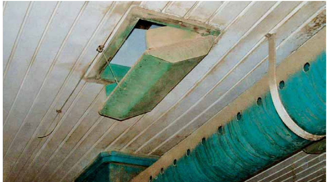
Correct adjustment of air inlets is essential to avoid drafts that can lead to tail biting
