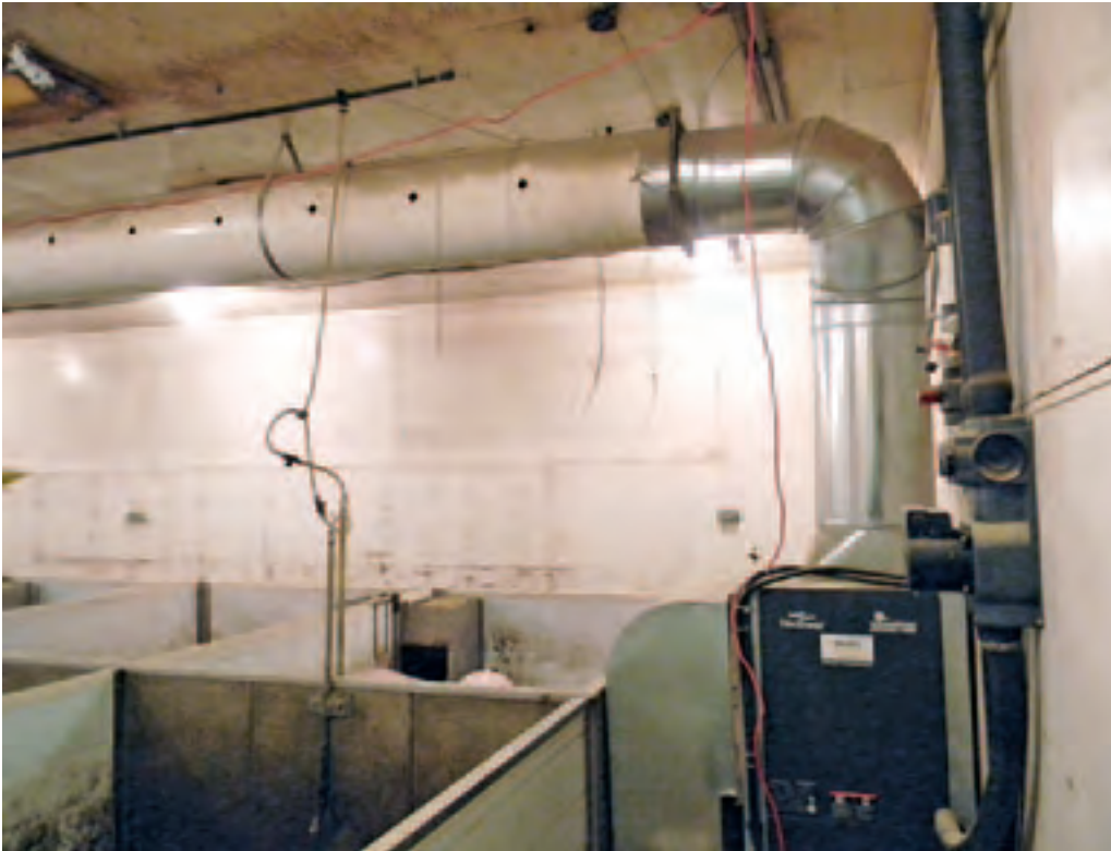
Using a heat pump unit resulted in a 52% reduction in energy consumption compared to a conventional forced-convection heater
