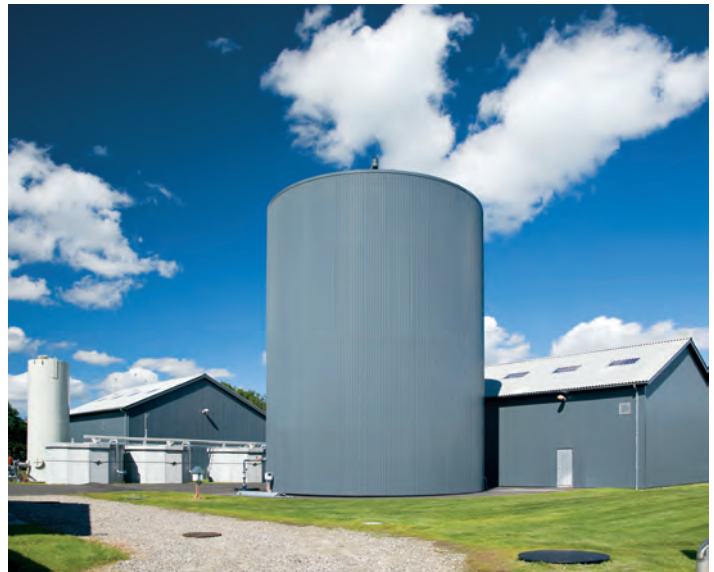
Biogas digesters are helping to reduce greenhouse gas emissions from Danish livestock production
