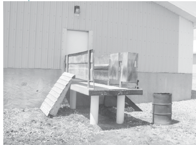
Figure 3. External loading ramp allows trucker to assist without entering barn. Note also the ramp extension used to reduce angle of truck ramp to top deck.
