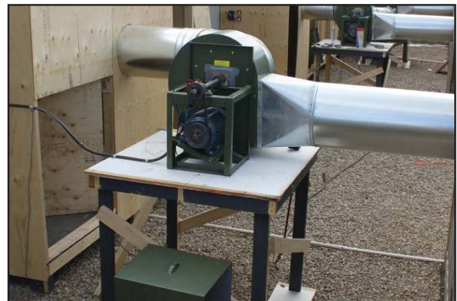
Figure 2. Actual installation of air cleaning unit at a grower finisher room
