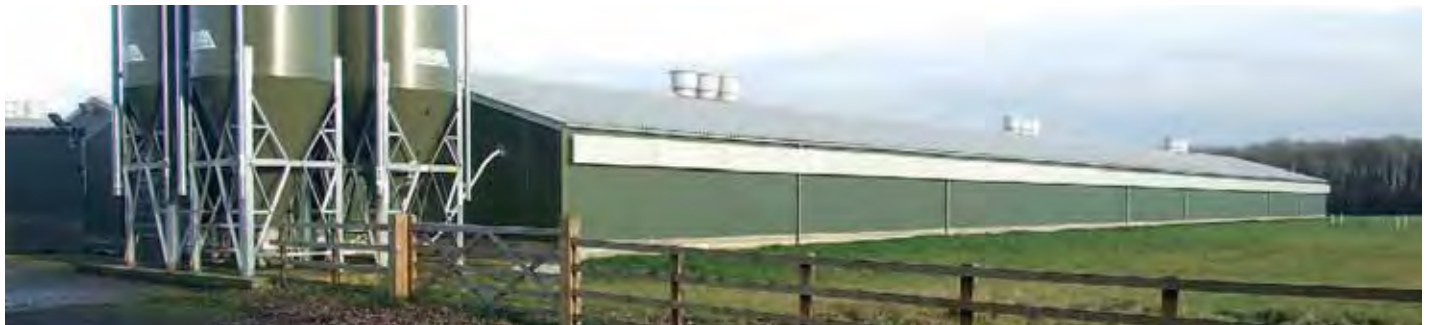
This new building is the result of 1.5 million GBP investment by JSR Genetics in East Yorkshire, UK. Photo by Stuart Lumb
