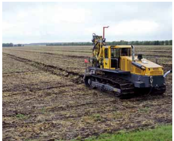
Tile drainage installation
