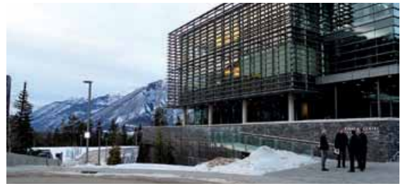
The Kinnear Centre for Creativity and Innovation has long been a part of the Banff Pork Seminar, but next year, the seminar is moving to the Fairmont Banff Springs Hotel.
