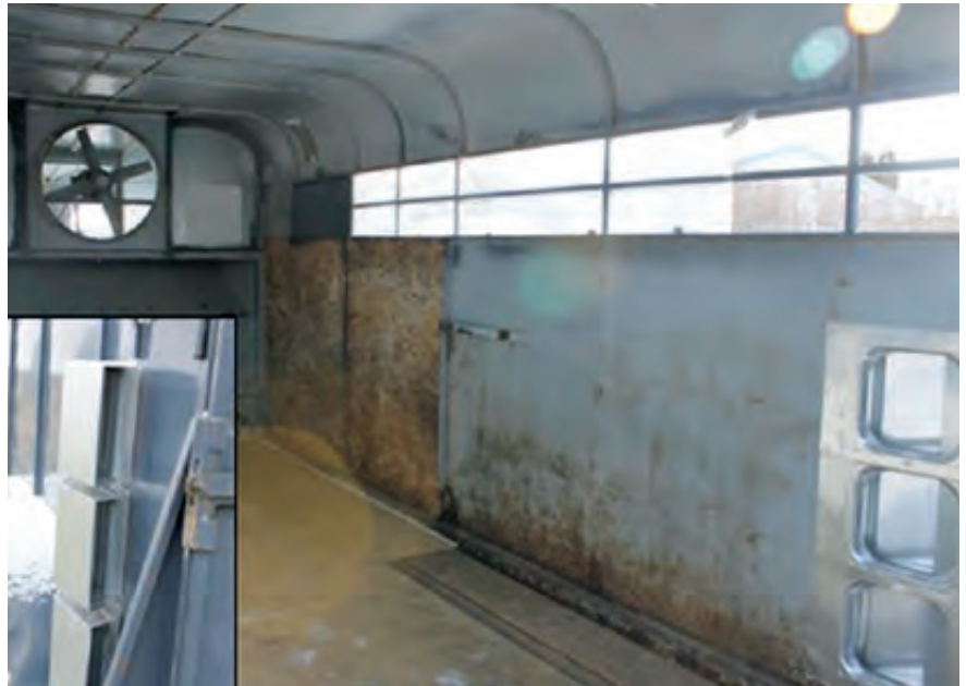
Figure 2. A ventilation fan and air filter holder were installed in the gooseneck area which was partitioned from the animal compartment of the trailer. Exhaust vents (inset) were installed on both sides of the trailer.
