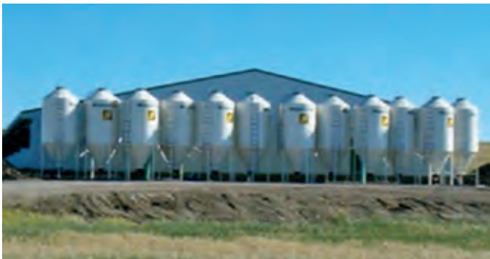
The Drumloche Research Barn has two rooms with a capacity to conduct two research trials simultaneously. Each room is serviced by six bins, each with an eight tonne capacity.
