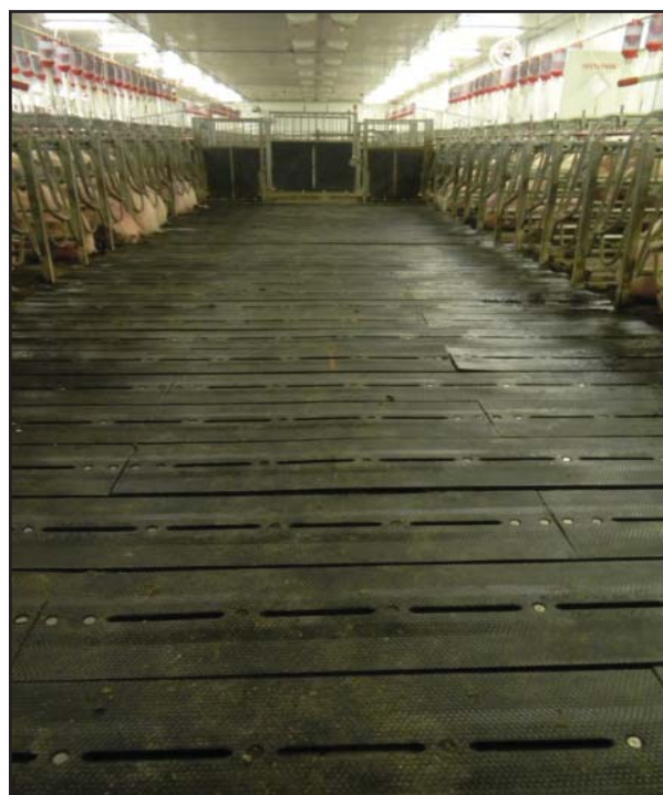
Figure 1. Rubber slats installed in an I-pen.
