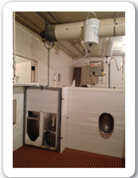
Figure 2. Modification with whey feeding buckets above the metabolism crates
