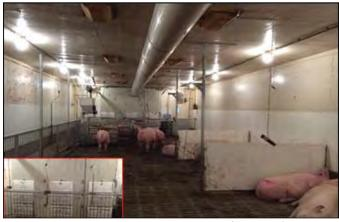
**Figure 1.** Photos of the control room with the existing (unmodified) ventilation system (A) and the treatment room with the air inlets on the opposite side (B) following the principle of a horizontal flow ventilation system. B – inset: wall air inlets installed in the treatment room.
