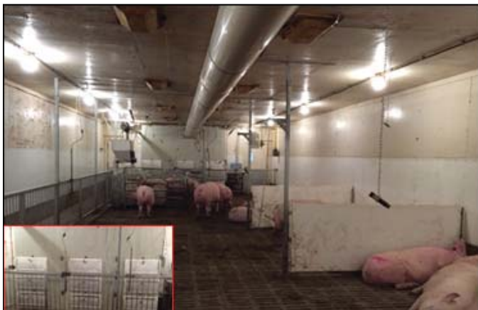
Figure 1. Photos of the control room with the existing (unmodified) ventilation system (A) and the treatment room with the air inlets on the opposite side (B) following the principle of a horizontal flow ventilation system. B – inset: wall air inlets installed in the treatment room.
