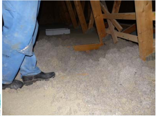
Ceiling, insulation, trusses and truss plates
