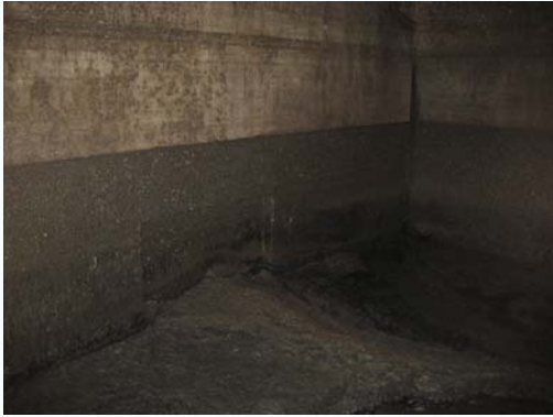
Footings, foundation wall, pit walls
