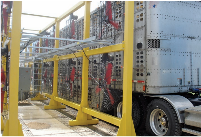
Ventilation system. Source: Sherbrooke Research and Development Centre, AAFC
