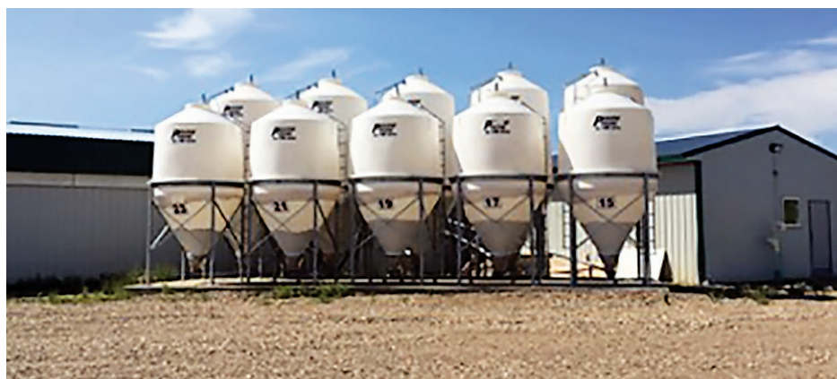
Front view of the Lewisville Nursery Research Barn. The barn is serviced by five smaller (four tonne) and five larger (six tonne) bins with the possibility of testing up to five experimental diets.
