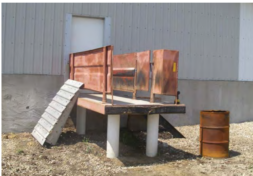
Figure 3. External loading ramp allows trucker to assist without entering barn. Note also the ramp extension (on the left) used to reduce the angle of internal truck ramp to the top deck
