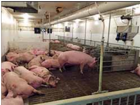
Photo of the control room with the existing (unmodified) ventilation system (A) and the treatment room with the air inlets on the opposite side (B) following the principle of a horizontal flow ventilation system.
