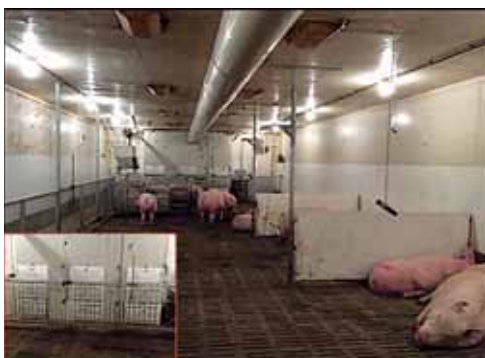
B inset – wall air inlets installed in the treatment room.
