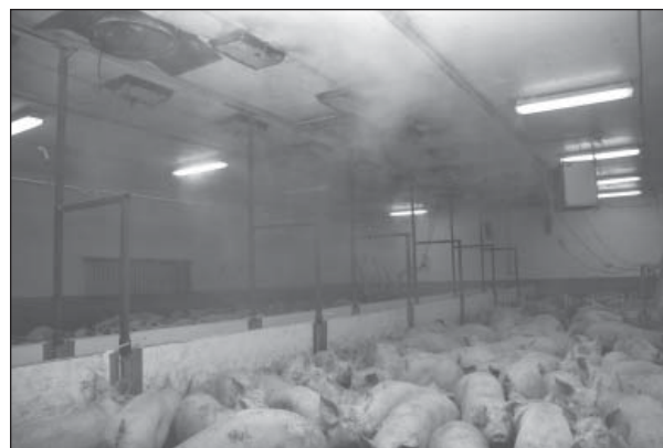
Over-ventilating a room by just 10% in the winter at current energy prices can cost producers an additional $3.00/hog marketed.
