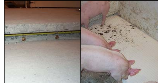
Figure 1. Water nozzles used to wash the manure from the gutter portion of the pen.
