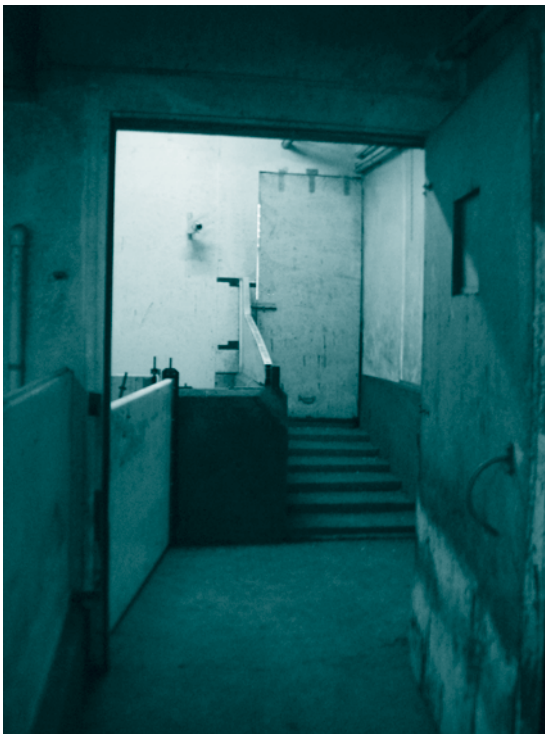
Figure 2. Well lit loadout with concrete steps (30 cm treads).
