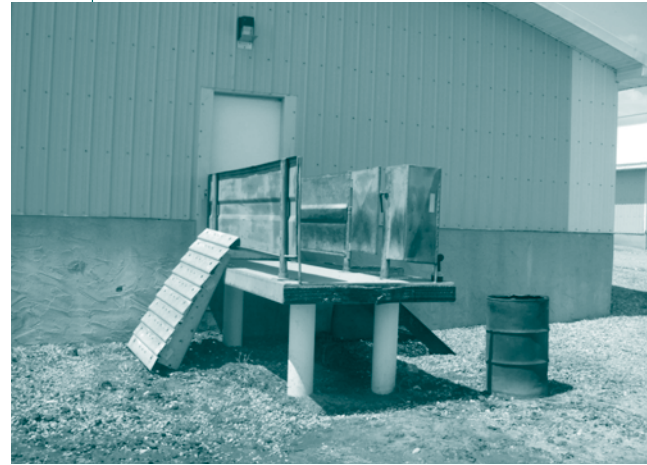
Figure 3. External loading ramp allows trucker to assist without entering barn. Note also the ramp extension used to reduce angle of truck ramp to top deck.
