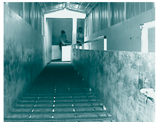
Figure 1. Hydraulic loading ramp with manway (looking down ramp from truck entry).
